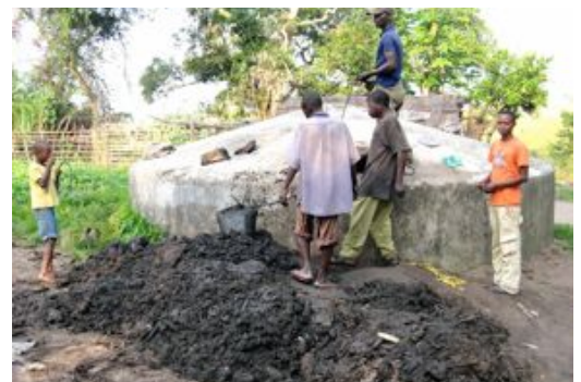
Cleaned out cistern.
